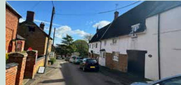
Figure 34: High level of enclosure created by 2-storey building frontages against a narrow street, High Street.
