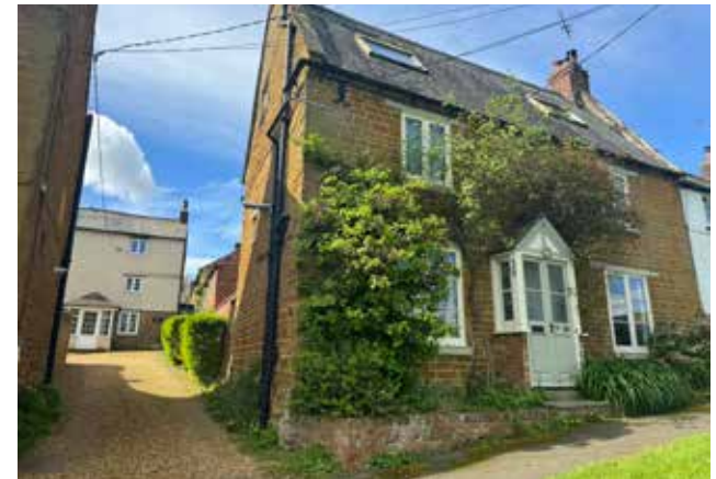
Figure 37: Example of back of plot infill in the historic core.
