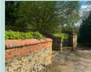
Figure 54: Low-rise brick and ironstone walls
