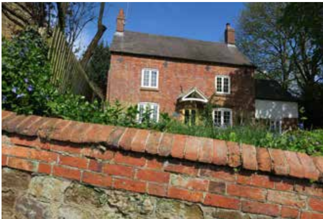
Figure 14: Example of red brick cladding in Flemish bond and brick and sandstone wall boundary with soft landscaping.
