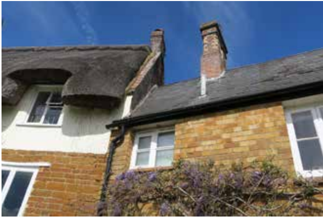
Figure 15: Example of Northampton ironstone and rendered walls with thatched and slate roofs.
