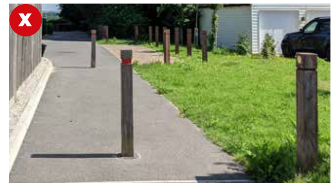
Figure 63: Example of poles positioned centrally on a narrow pavement which obstruct pedestrian and cycling movements, which should be avoided, example from outside the parish.
